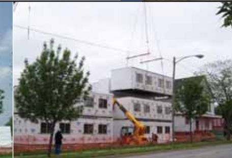
Day 35, Module Installation
