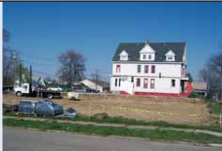
Day 0, Site Clearing
