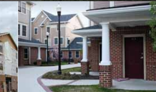
Day 120, Project Completion
